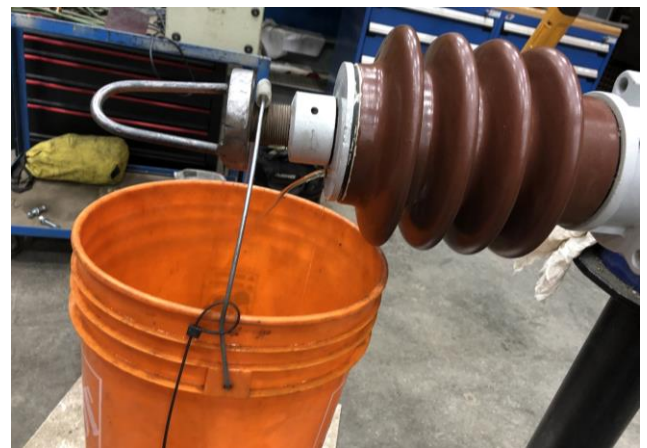
Fig 7 – Drain oil from bushing
