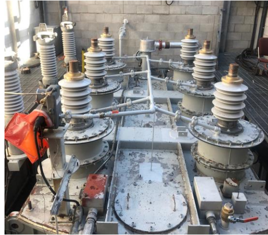
Fig 2 – Bushings installed on a transformer.
