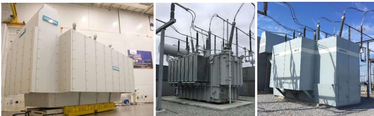
Figure 7 – Bullet resistant transformers – new and retrofit solution (photo: Siemens)
