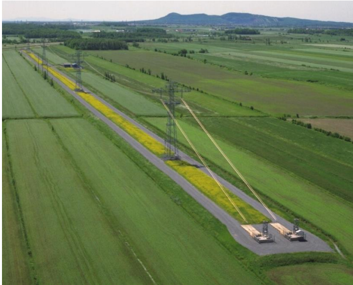
Figure 6 IREQ's test line
