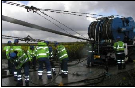
Fig. 2. Mid-span joint replacement operation
