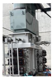
Figure 3- External connection box to connect the single phase transformers to bank configuration
