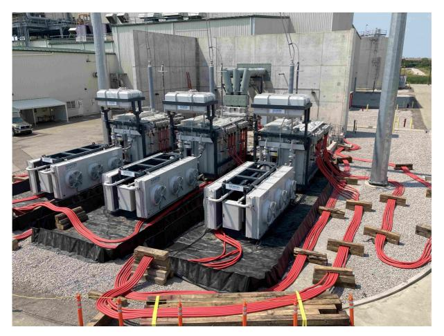
Figure 5 – 250 MVA bank – 345 kV Pretact<sup>™</sup> Resilience Generator Step-Up Transformers On site – Completely installed and energized
