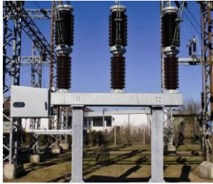
72.5 kV Blue Circuit Breakers, LT 6 in operation in EU since 2010 2 in operation in USA since 2020
