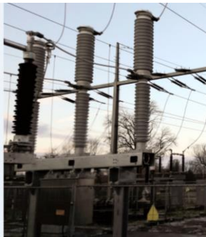
145 kV Blue Circuit Breakers, LT >150 ordered for GER, POL, NOR, SWE, DEN, KAZ, USA, CHE, GBR, ROU... Thereof >100 in operation,
