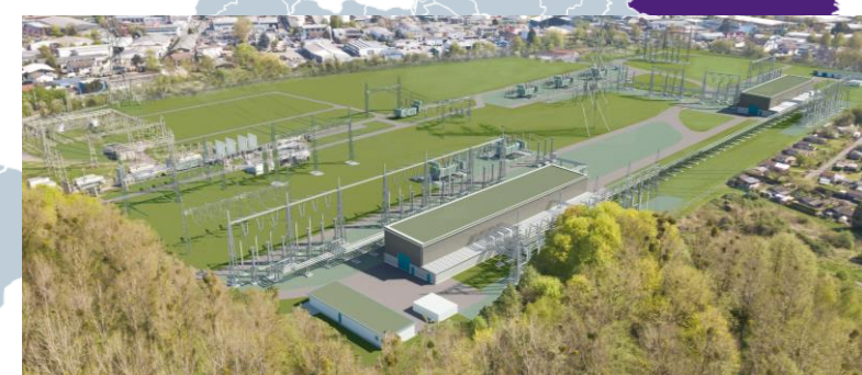
420 kV Blue GIB, extensions, bushings >5000 m single-phase ordered in GER, 600 m delivered GBR
